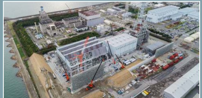
T-Point 2 during construction, October 2019.
