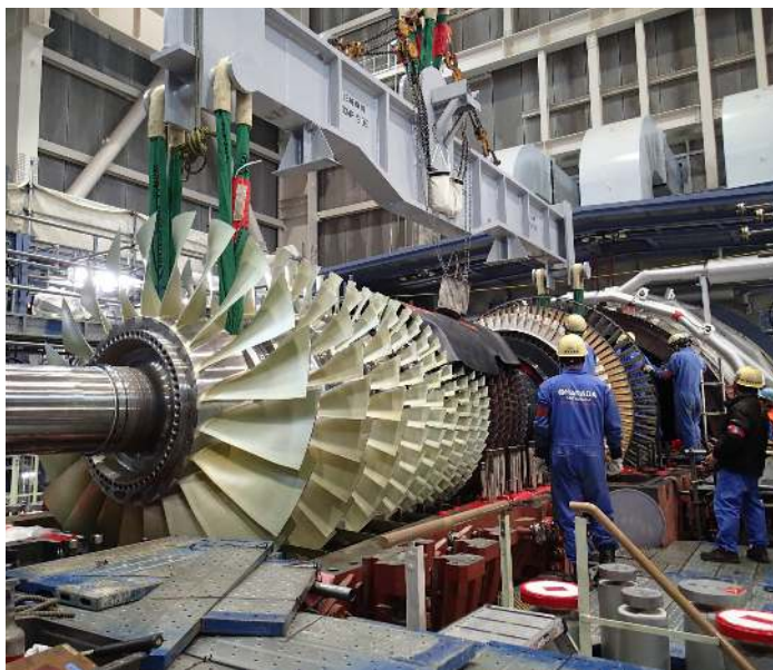
M501JAC rotor installation.
