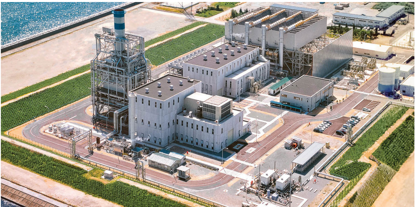
Grid-connected validation plant, T-Point. Hyogo Prefecture, Japan
